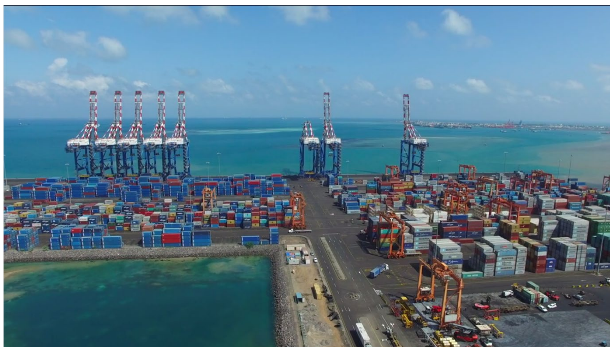
Figure 11.1: Aerial view of SGTD (prior to the installation of the mega-max STS Gantries)
